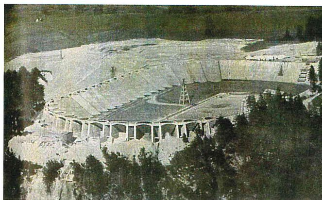
Figure 8. General view of Rutte dam
