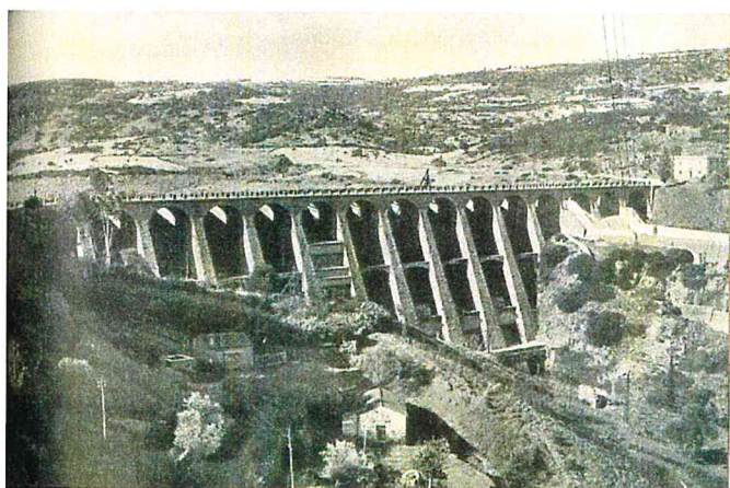
Figure 6. Downstream view of Santa Chiara dam
