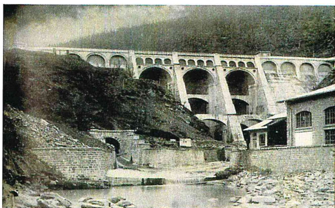
Figure 5. Downstream view of Pavana dam
